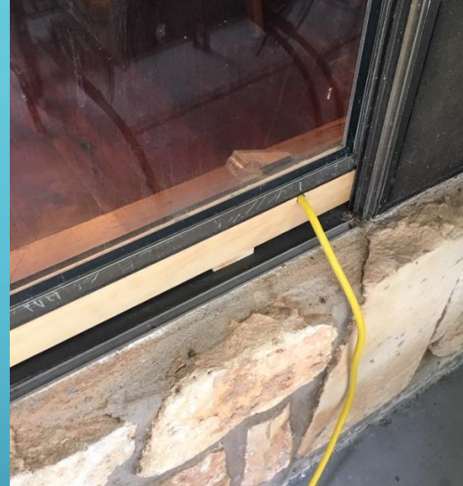
Cut the board To fit the window
